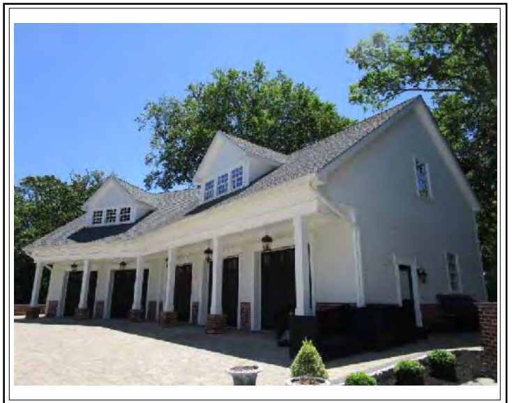
5/Car Detached Garage - Front Photo #2
