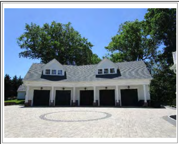
5/Car Detached Garage - Front Photo #1
